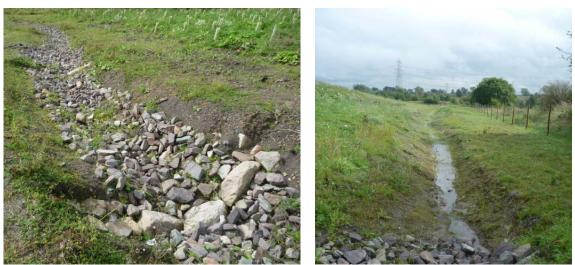
**Figure 11.** South-west tip, armoured drain with sill (left) and merging into swale on west boundary (right) on 9/9/11
