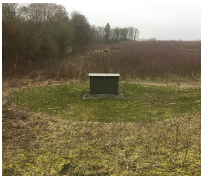
Tree planting around three boreholes to improve and protect the groundwater supply for a small town in Denmark as part of a PESFOR-W scheme.
